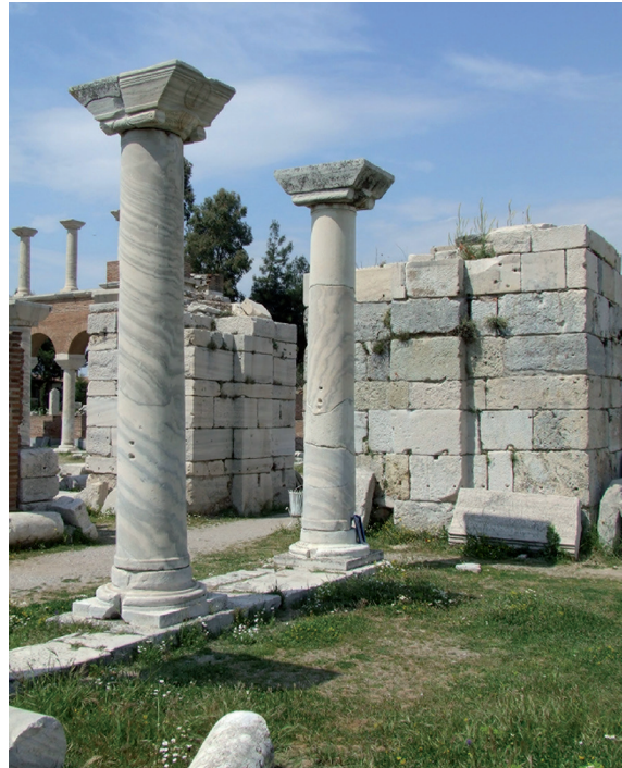
14 View of piers showing the constructional difference between the piers of the transept (right) and the piers of the nave (left). The piers of the transept are made of courses of similar heights, whereas the piers of the nave are built with an alternation of thin and thick courses
