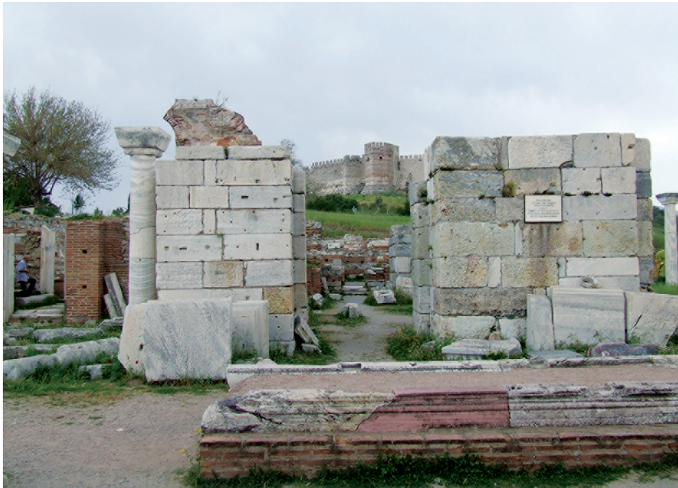
15 Detail of the ›redundant‹ pilasters between the piers of the crossing and the piers in the east extremity of the nave
