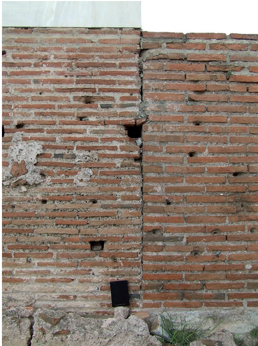
13 Detail of the vertical joint between the external walls of the nave and the transept
