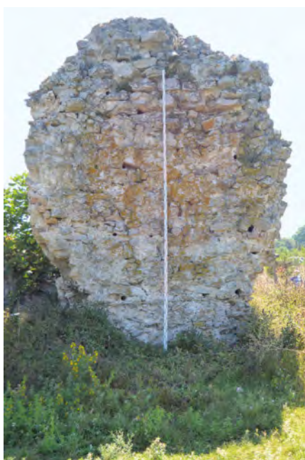
17 Wall no. 4, rows of cut stones
