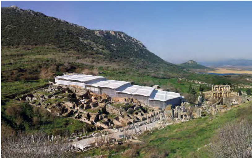
2 View of the roofed Terrace House 2 and Terrace House 1 in front
