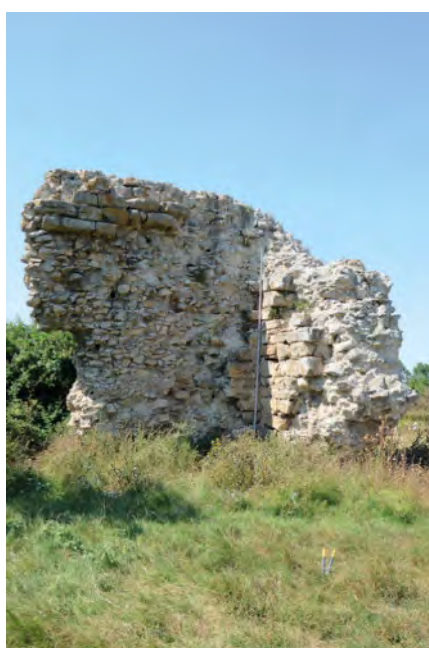
18 a Wall no. 5, east side
