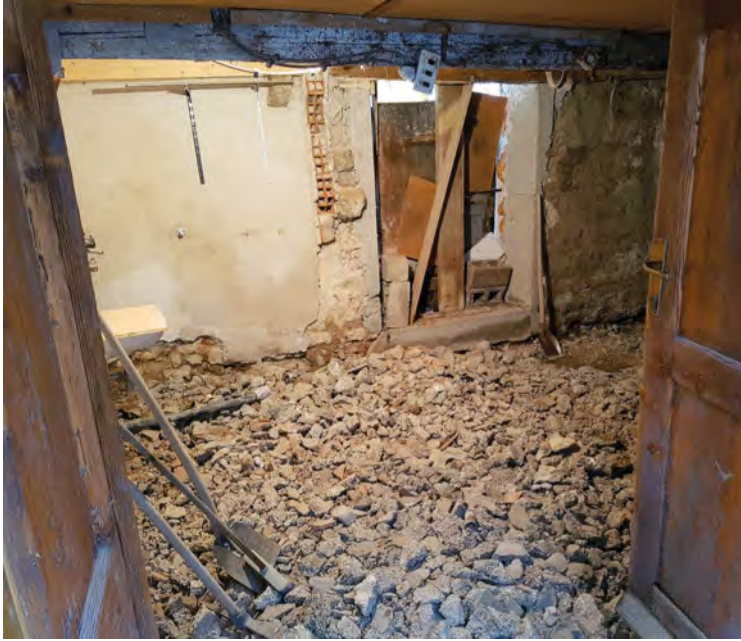
5 Trench 1/18. Removal of concrete floor in the basement
