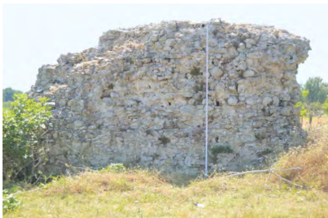
16 a Wall no. 2, east side
