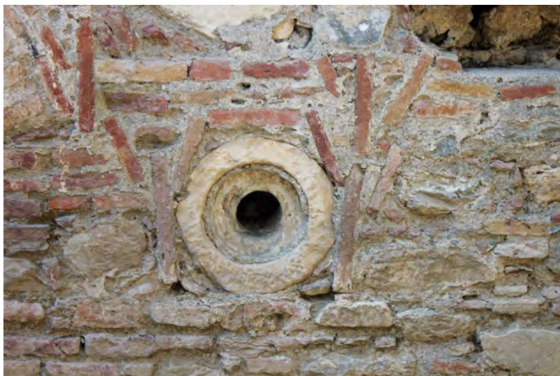
10 Decorative use of bricks on the wall of the Türbe in the Artemision (© OeAW-OeAI, E. S. Bellibaş)
