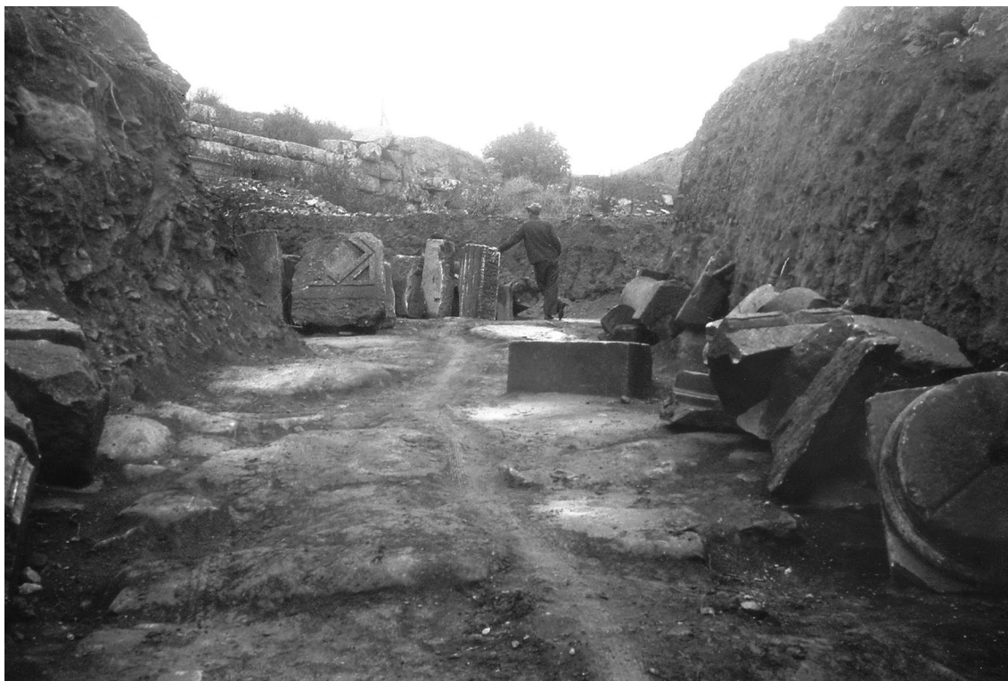
5 Miltner's excavation of the Curetes Street (© OeAW-OeAI, Archive)
